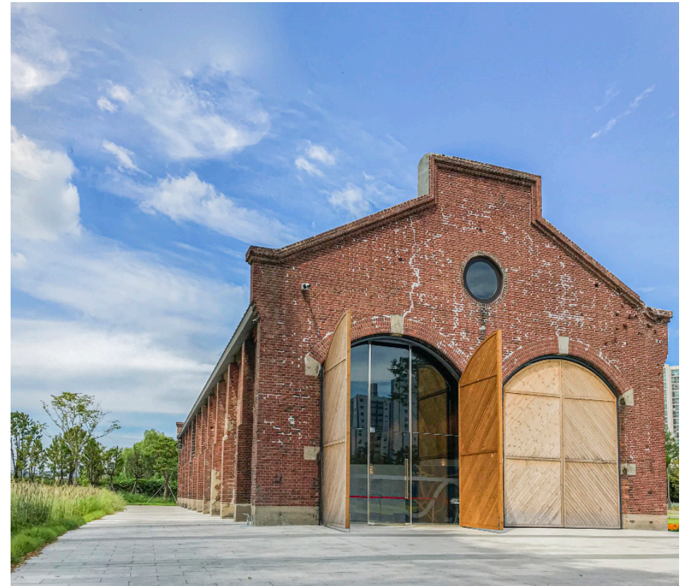
Vehicle Maintenance Depot at Jinju Station
